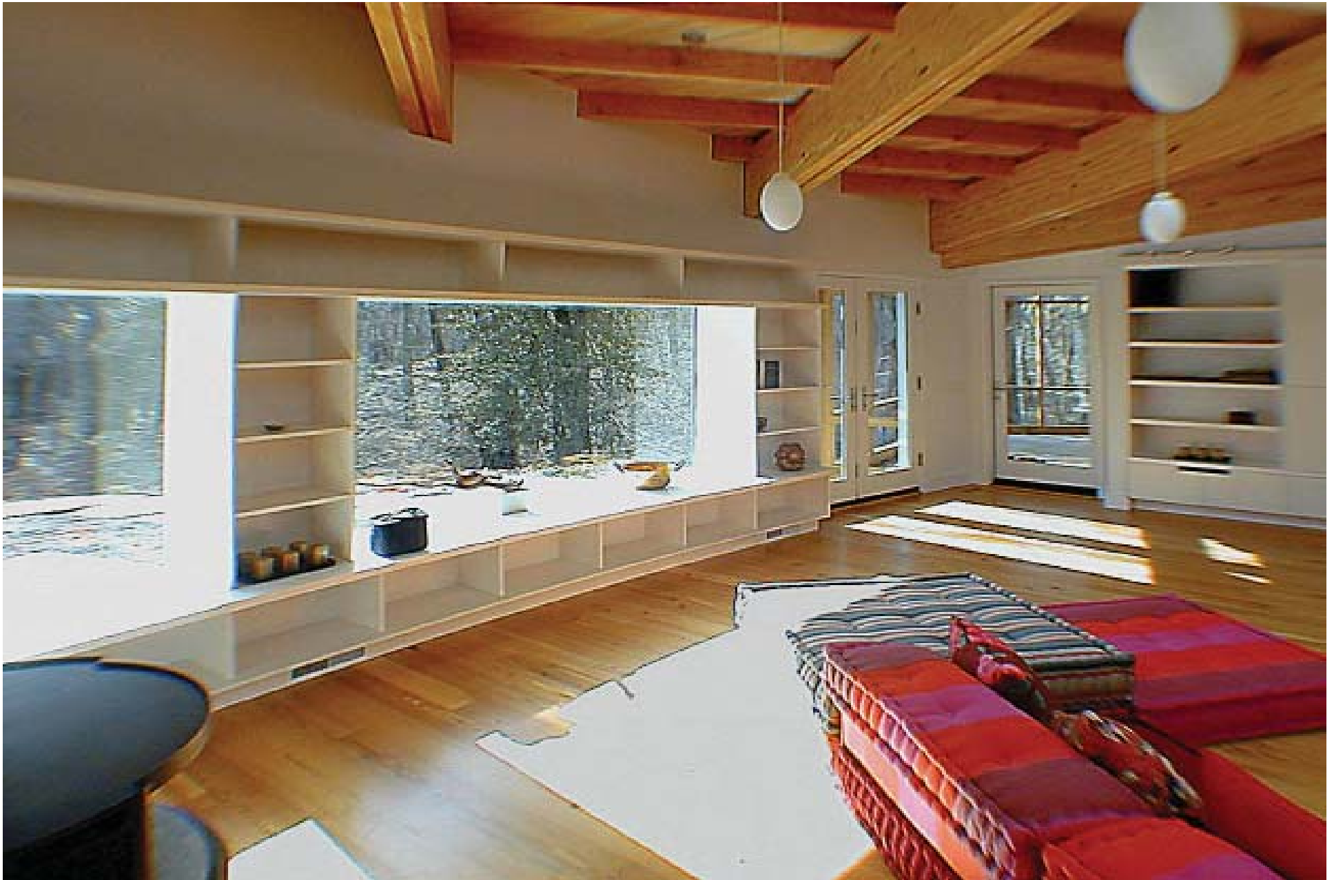
9. LIVING ROOM- View of southerly exterior wall showing desired light penetration in the winter time. Exterior overhang protects in the summer time.
