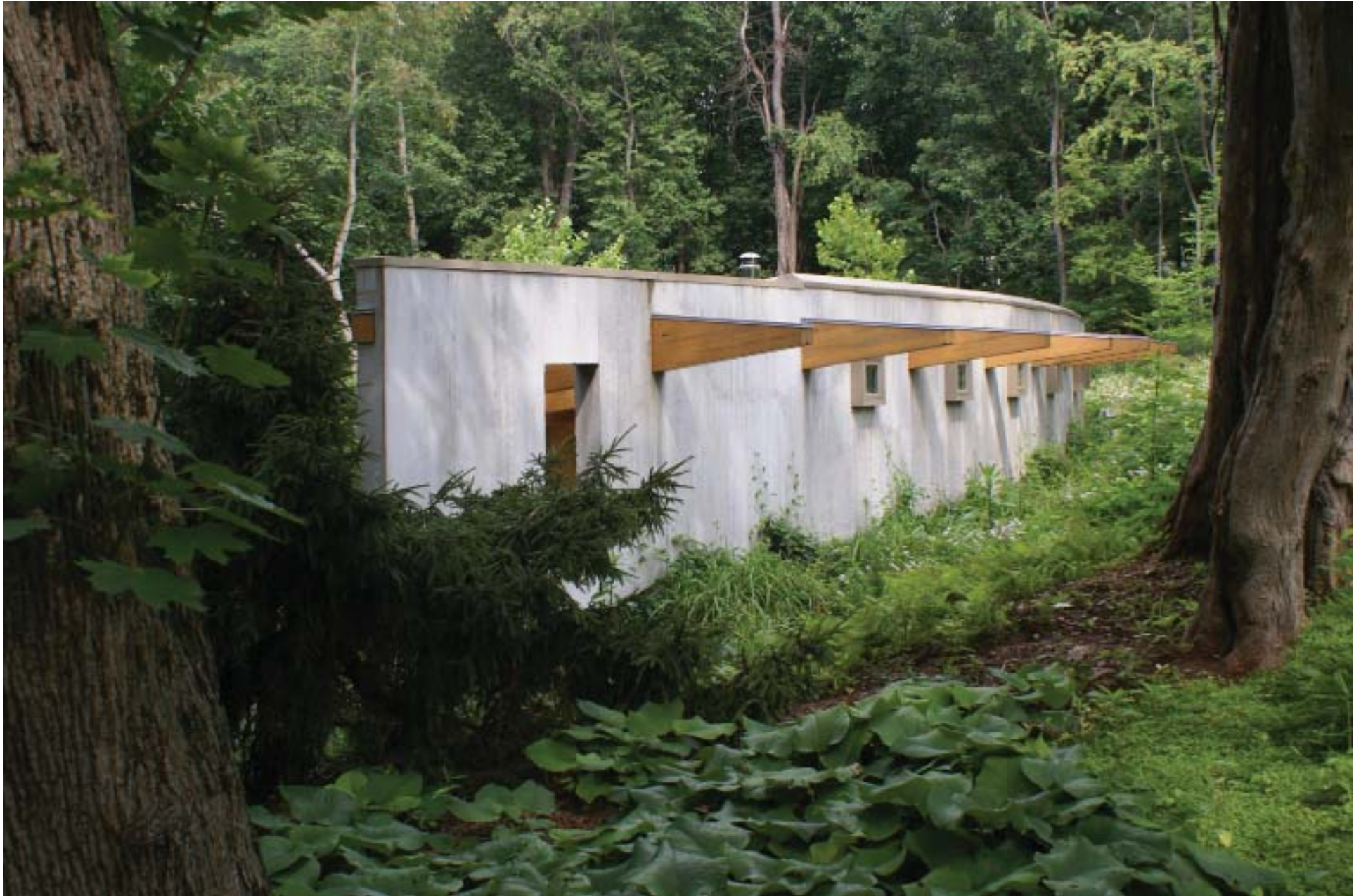
11. EXTERIOR- View of curved retaining wall with beam projections showing.
