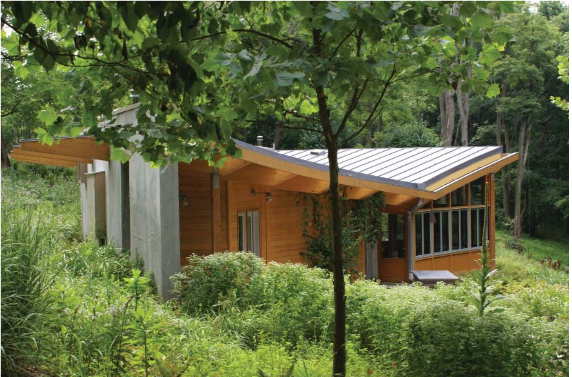
10. EXTERIOR- View of West end of structure standing on cart path. Curved retaining wall is on the left, exterior wall of painting studio is on the right.
