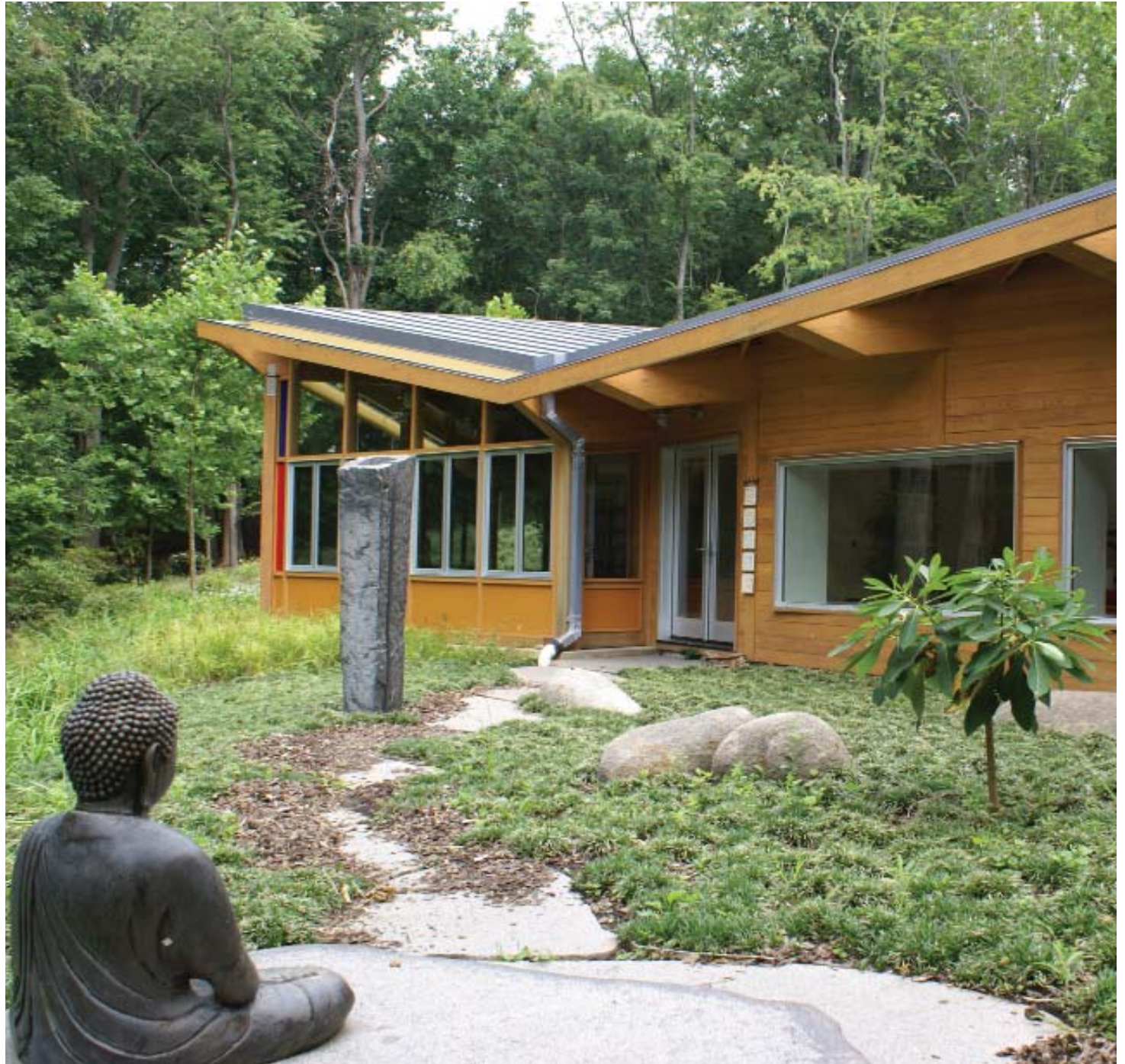
8. APPROACH PATH- Shows partial view of South elevation, granite sculpture & stepping stones. All season porch is on left behind sculpture. Wall of living area is on right.
